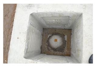
After the mortar is hardened around the foundation connector, the column can be installed.
